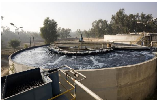
Fig. 15. Aerobic oxidation tank
